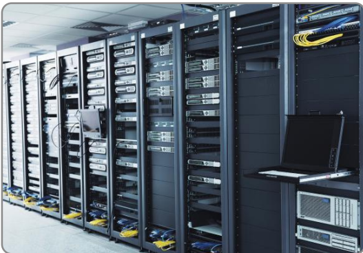
Enterprise Cabling & Security Solutions
